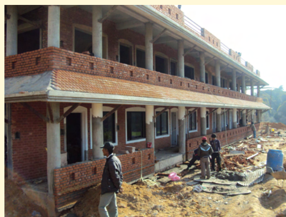
Tewa Dormitory building under construction
