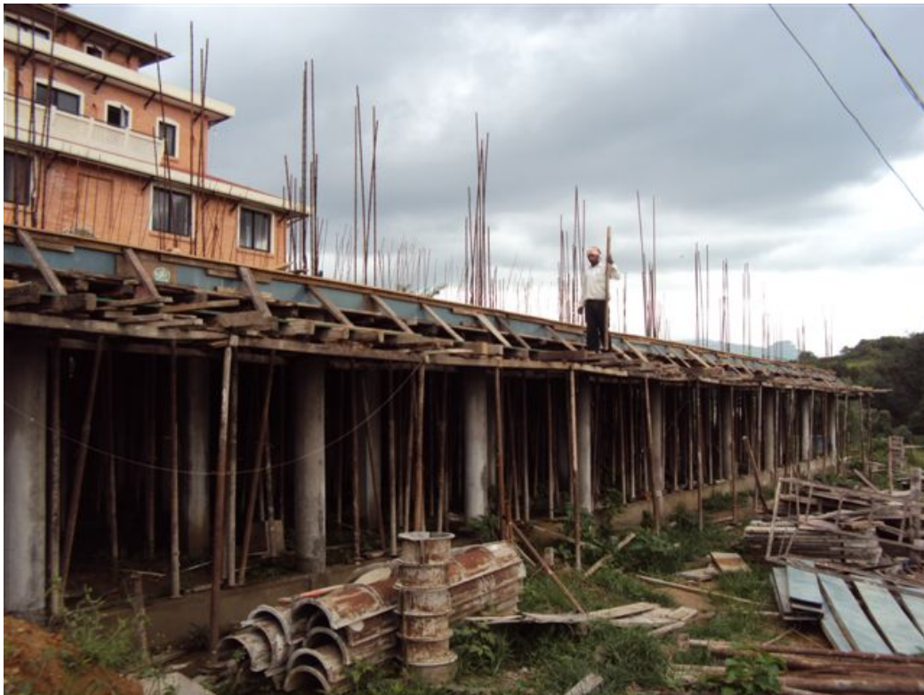
Looks messy now - but there is much work to it!
