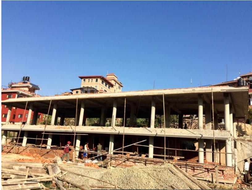
We can see that the skeletal of the A3 is ready. Brickwork on the ground floor is also finished. After the Tihar holidays the brickwork will move to the first floor and terrace. Then the plaster, plumbing and electric work will begin. After the initial glitches in availability of raw materials, work is moving smoothly.
