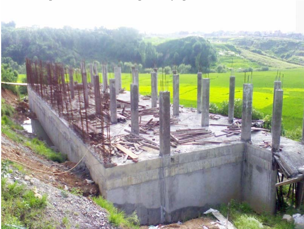
Columns for the Dormitory Second Floor!
