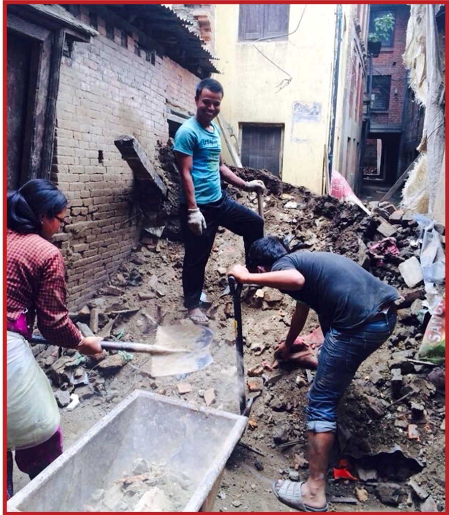
Clearing rubbles with a smile
